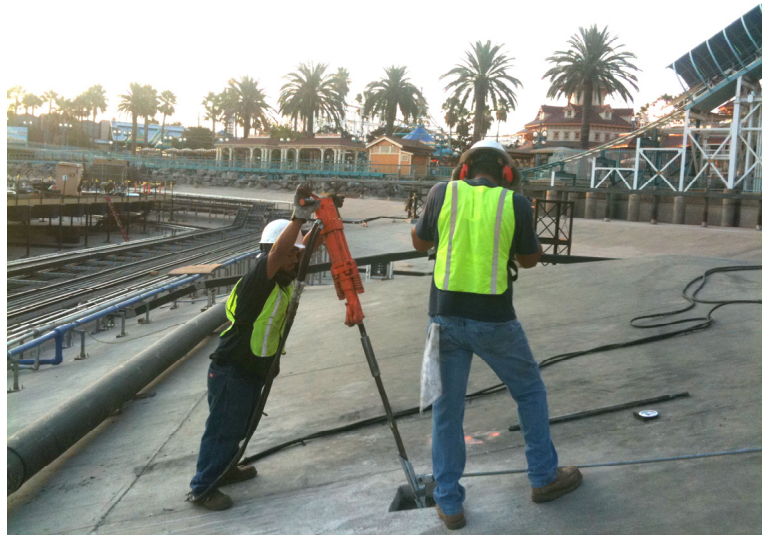
Fig. 19-1 – Installing an Earth Anchor. Earth anchors can be an effective and space efficient alternative to using bulk weight to ballast structures and rigging.
