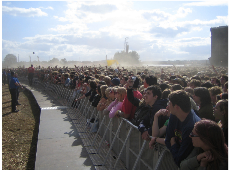
Fig. 23-6 - A standard concert stage barrier, note the diagonal bracing stays which allow the barrier to resist horizontal load. Note also the extended rear plate allowing security personnel easy access and a safe platform from which to assist or rescue the public. Photo courtesy of The Event Safety Shop, LTD.
