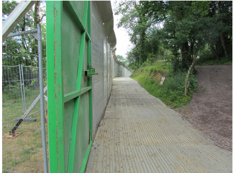
Fig. 23-5 - A custom-made fence designed to create an impregnable event perimeter. Block and mesh panels form an inner fence to create a moat in which security can operate.. Photo courtesy of The Event Safety Shop, LTD.
