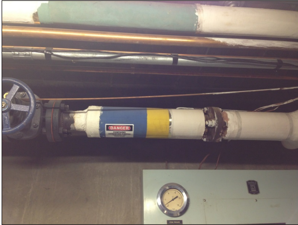
Photo 3: Warning label on asbestos straight-pipe insulation in boiler room.
