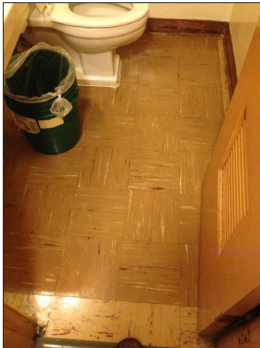
Photo 6: 9-inch Vinyl Floor Tile (VFT) in small restroom.
