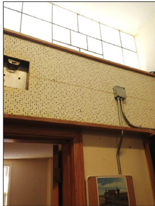
Photo 10: Fiberboard found to have non-asbestos adhesive.
