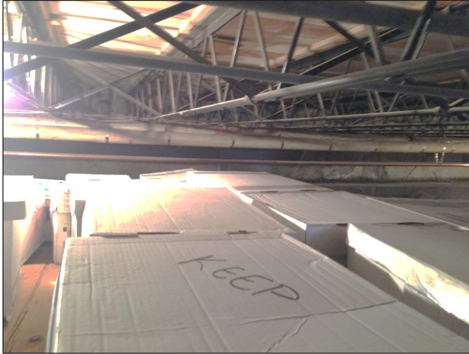
Photo 7: Storage space under stage with asbestos straight-pipe insulation. Approximately four pipes are present in fair condition. Folding chairs and files are stored in the room.
