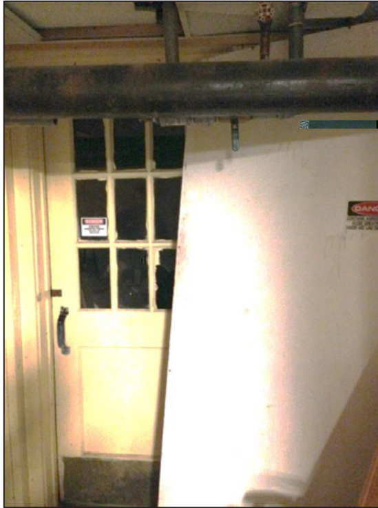
Photo 5: Door to the pipe corridor. Asbestos warning labels on doors.
