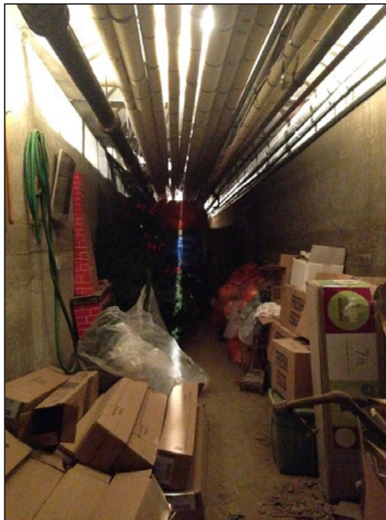
Photo 4: Interior pipe corridor with approximately 12 straight pipes of various sizes (2 to 6 inches). Asbestos insulation is in fair condition.
