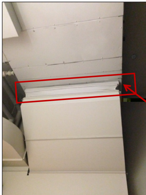
Photo 8: Vibration collar on heating unit in stage/gymnasium area. Sample not collected during this investigation, and the material is assumed to contain asbestos.
