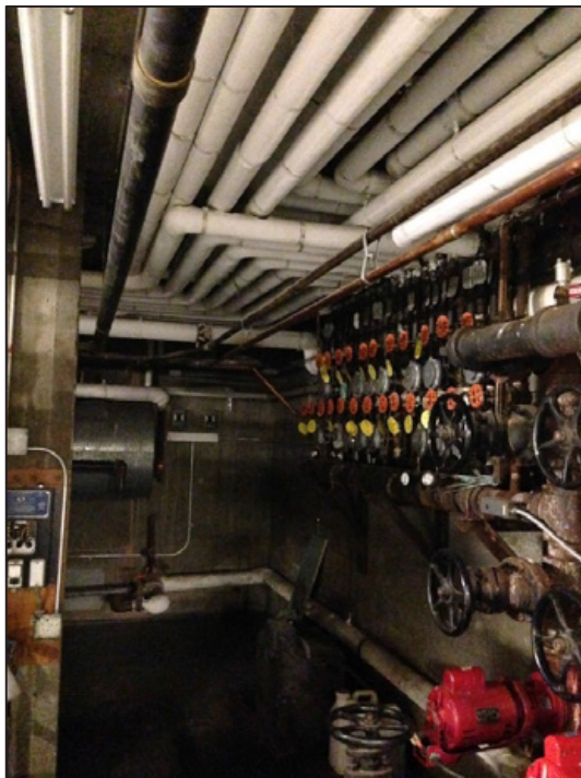
Photo 2: Boiler room with asbestos straight-pipe insulation. Approximately 20 insulated lines are shown.
