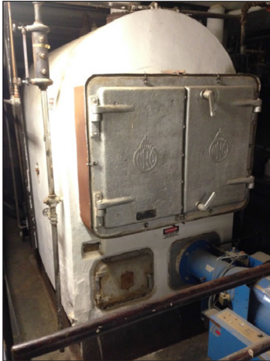
Photo 1: Boiler in basement. Asbestos caution labels on exterior of boiler. Asbestos in good condition.
