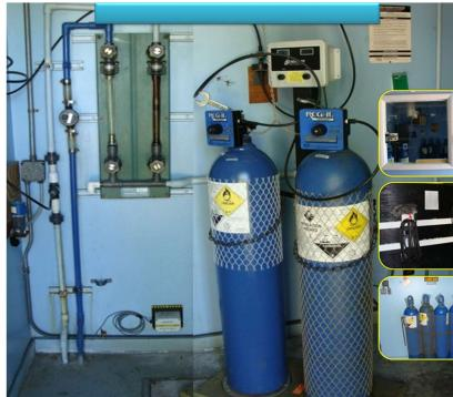
serious incident А occurred in 2018 when heater control a (thermostat) would not shut off the heater. The heater control had corroded, and there was no alarm. As the temperature in the room rose, the gas within the tanks rose in pressure and a leak occurred. When an operator opened the door he was hit with the gas and had to go to the hospital. Не was later releases, but the city realized
