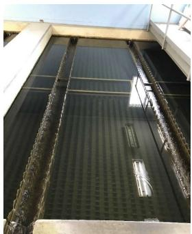
Figure 2-30 Forsyth Tube Settlers
