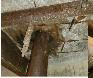
Figures ES-1, 2 Advanced Corrosion to Intake Floor Supports
