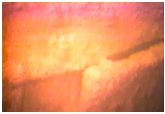
Figure 2-17 14-inch Intake Line Damaged and Offset Joint
