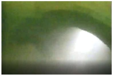
Figure 4-5 Intake Pipe Inlet in Good Condition
