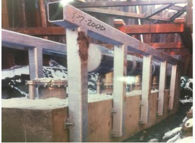
Figure 4-8 Johnson Screens and Support Used in Glendive
