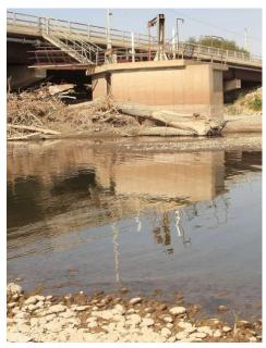
Figure 4-13 Defunct Crib and Barrel System in Laurel
