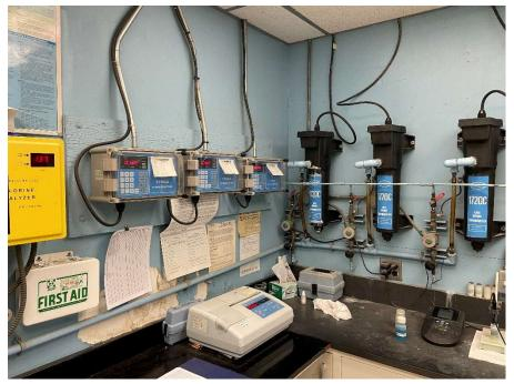
Figure 2-31 Turbidity Meters and Continuous Chlorine Monitoring
