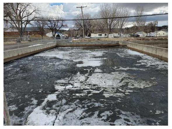
Figure 2-33 Backwash Settling Basins
