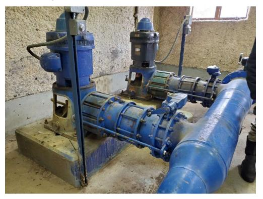
Figure 2-25 Low RPM Vertical Turbine Pumps at the Intake
