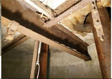
Figure ES-3 (Right)–Precarious Lower Level Suspended from Floor Above
