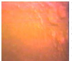
Figure 2-18 Tuberculation from Corrosion of 14-inch Intake Pipe
