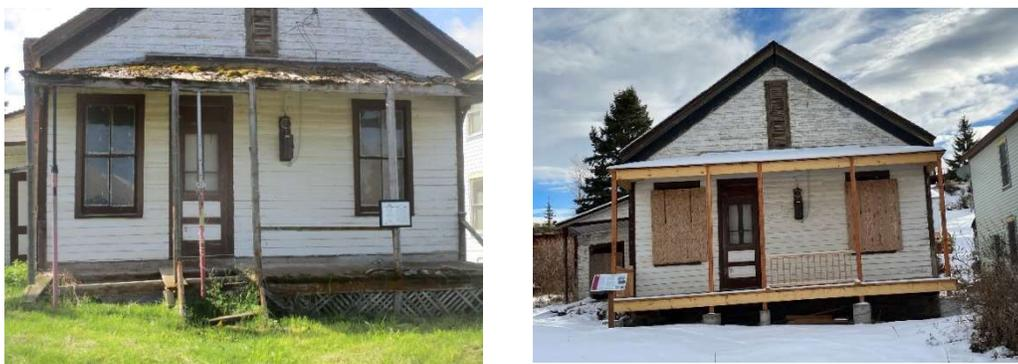
Hickman House masonry foundation and front porch stabilized – before and after (2023)
